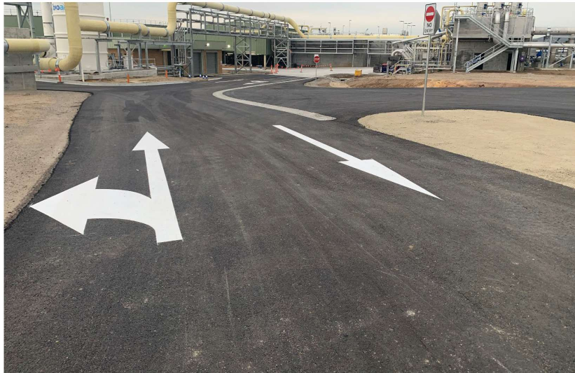
Sitewide signage, line marking, and spoon drains completed
