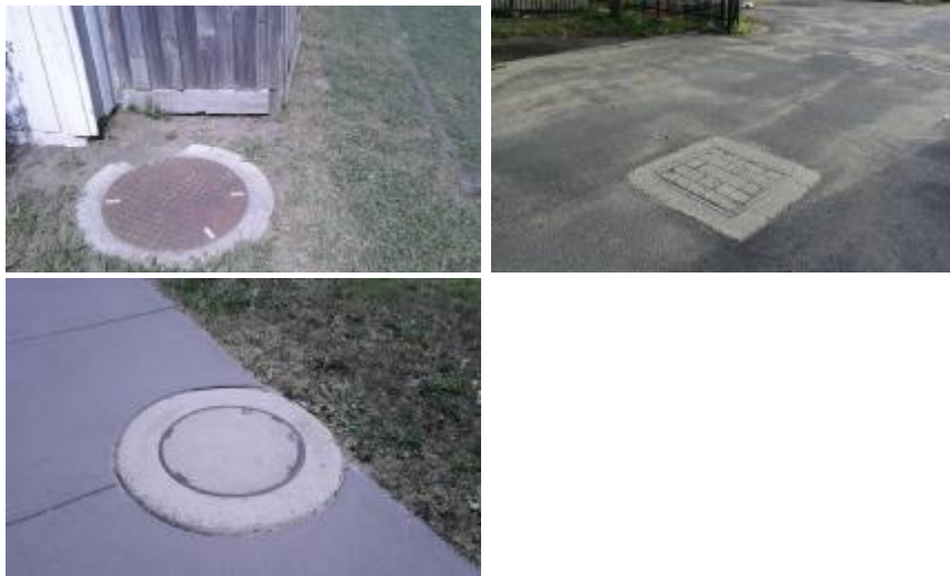
Figure 25- Maintenance holes
