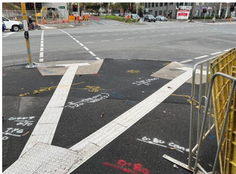
Figure 1: Paints used to mark underground services on a South East Water project
