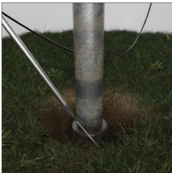
Figure 2: Two images showing the potholing technique
