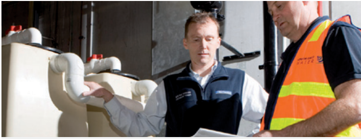
Test water is recirculated through the newly installed tanks.
